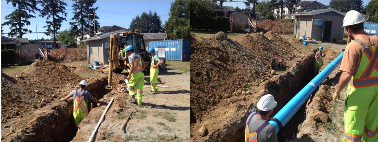
IMAGE | FURTHER TIE-IN CONSTRUCTION WORK FOR RW 2-63/17
