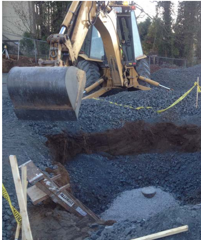
IMAGE | PERMANENT DECOMMISSIONING WELL 5-78
