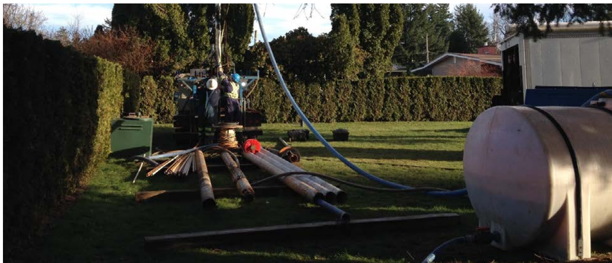
IMAGE | WELL PREVENTIVE MAINTENANCE – WELL FLUSHING FOLLOWING CHEMICAL TREATMENT
