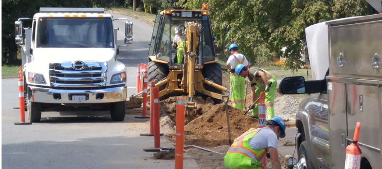
IMAGE | WATER MAIN UPGRADING WORK
