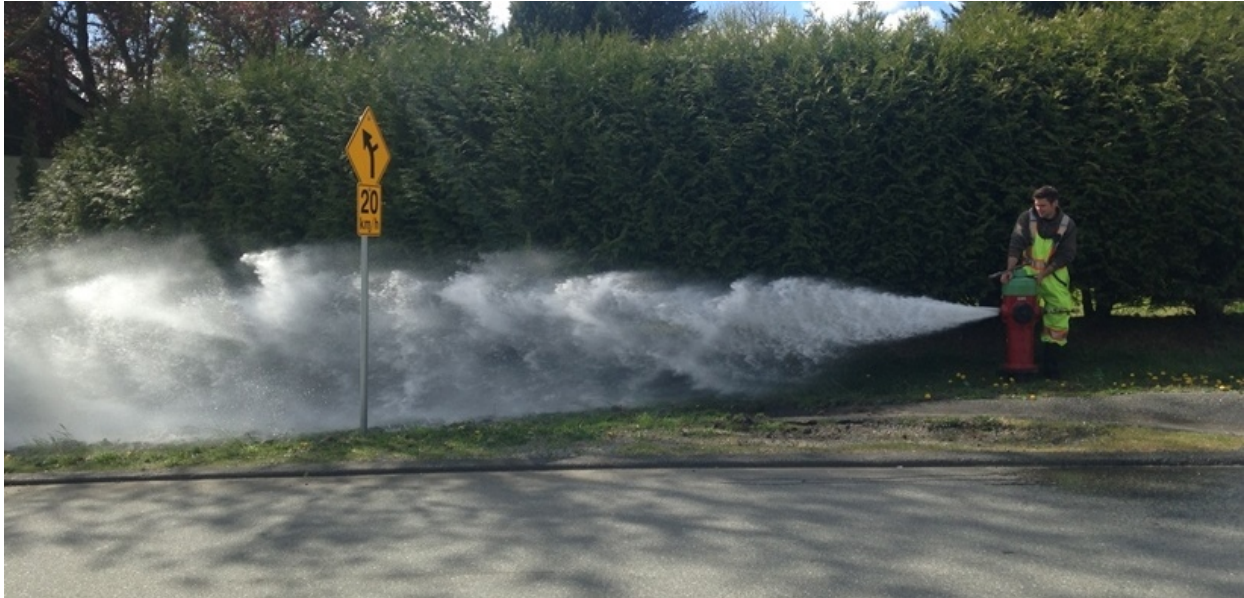
IMAGE | WATER SYSTEM FLUSHING VIA HYDRANT
