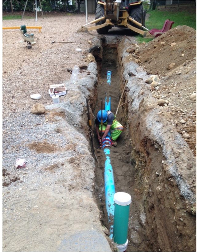
IMAGE | WATER MAIN REPLACEMENT
