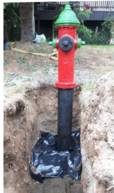
IMAGE | FIRE HYDRANT INSTALLATION
