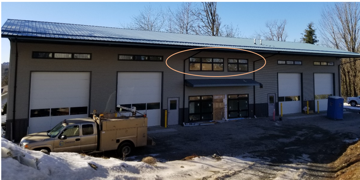
IMAGE | THE NEW OFFICE AT THE OPERATIONS FACILITY.
