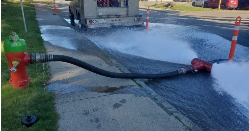
IMAGE | WATER SYSTEM FLUSHING IN PROGRESS.
