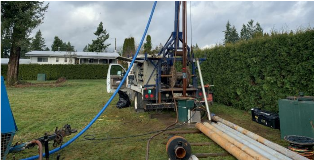
IMAGE | WELL REHABILITATION FIELD SETUP.
