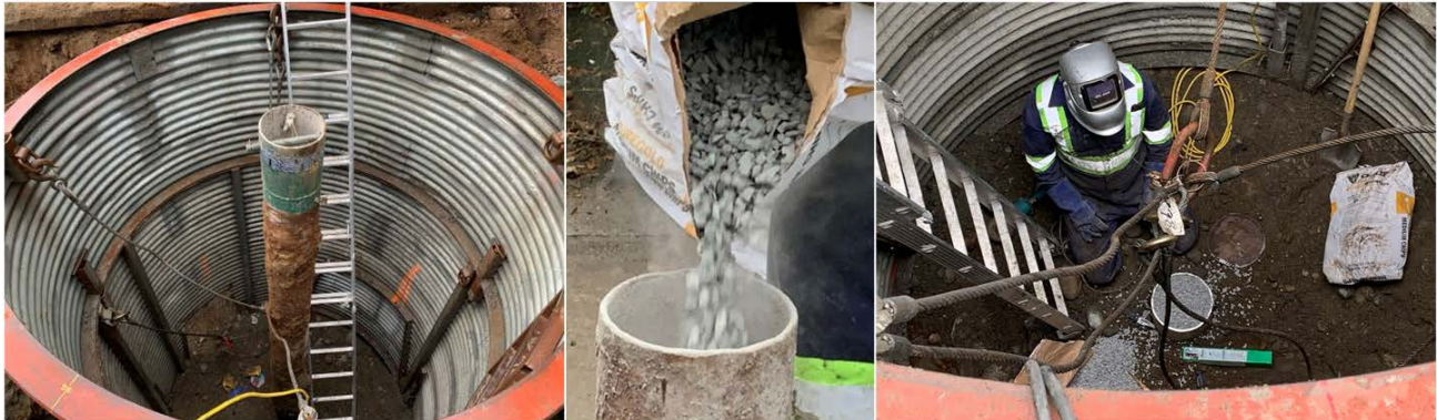
IMAGE | WELL CLOSURE WORK IN PROGRESS
