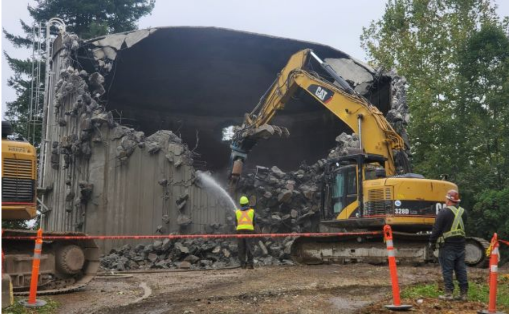
IMAGE | THE DEMOLITION OF RESERVOIR B COMMENCED ON OCTOBER 15, 2020.
