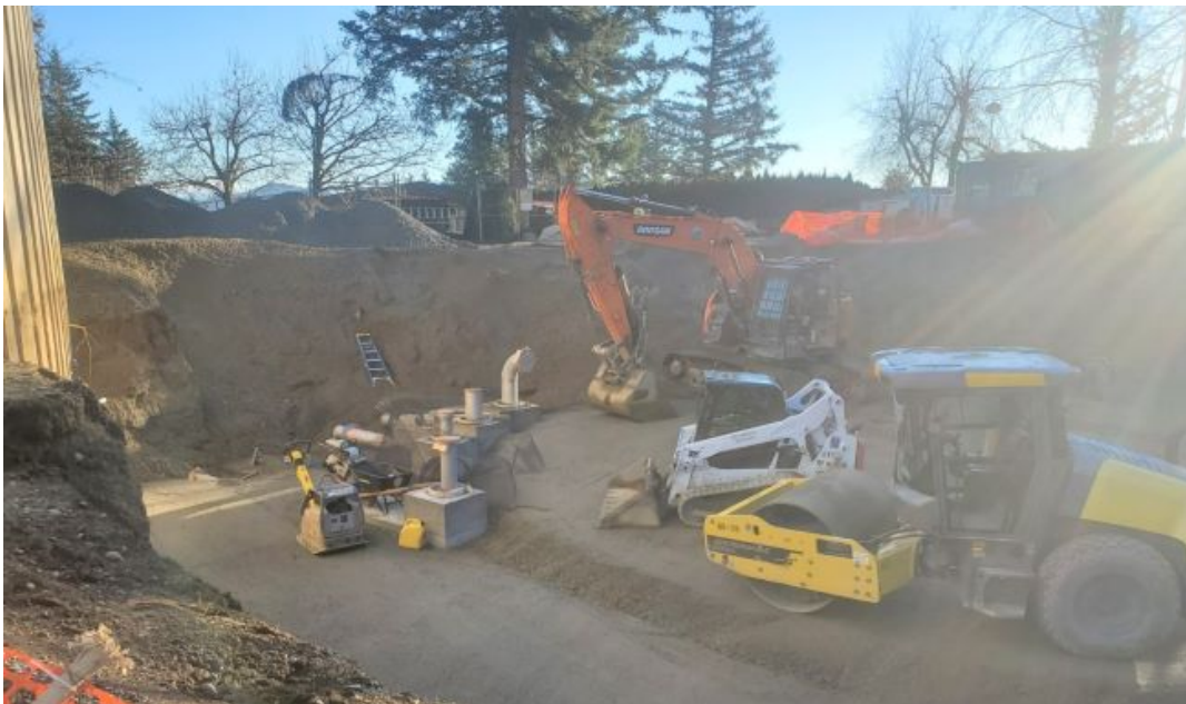
IMAGE | EXCAVATION WORK IN PROGRESS FOR THE NEW RESERVOIR (JANUARY 18, 2021).
